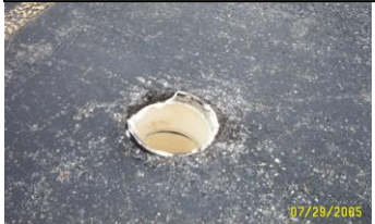
Repair or replace sewer cleanout covers!!
