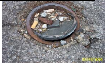
Repair or replace sewer cleanout covers!!
