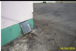
Repair or replace sewer cleanout covers!!
